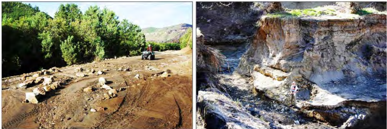
Figure 9. Flood impacts in East Canyon. Image to left shows debris covering Road 46; image to right shows new 25-foot deep gulley at the lower end of East Canyon (note person for scale)
